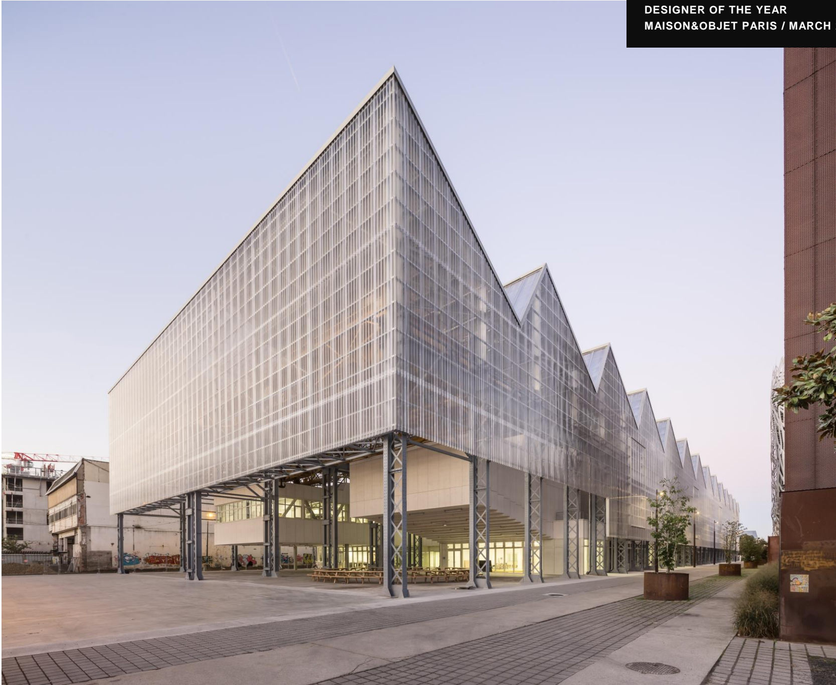
Franklin Azzi Architecture, Halles Alstom, ESBANM, Nantes, 2017 © Luc Boegly
