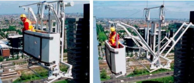
Top: Facade Access Strategy Plan Middle: Indicative BMU Bottom: Counterweighted Cradle for accessing set back facade areas
