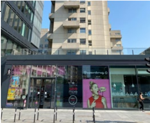
View looking north towards Kings Reach Building on Stamford Street. New retail activation on Stamford Street.
