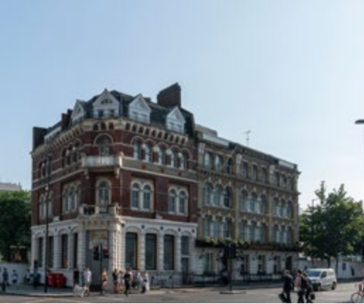
View looking south at 1 and 3-7 Stamford Street. Both are Listed Buildings and will be carefully considered throughout the design process.
