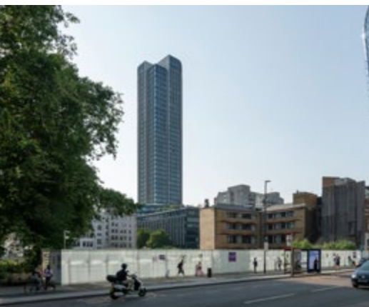
View looking north-west towards the Site from 240 Blackfriars Road showing a large portion of un-activated street frontage.
