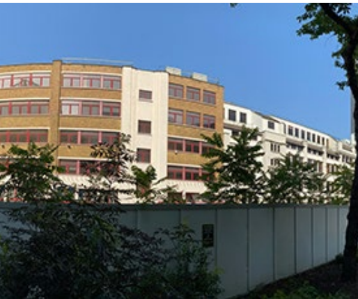
View looking West from the Site towards Paris Garden, with the a part of the former Clay's Printing Works visible.
