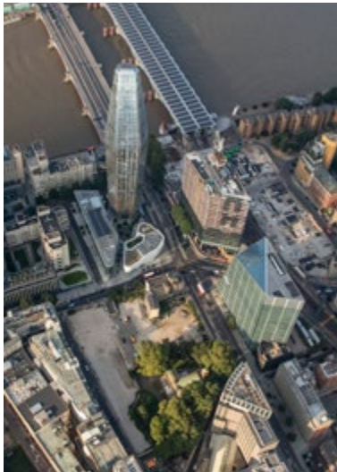
Current Site: Empty brownfield site in an exceptional central location.
