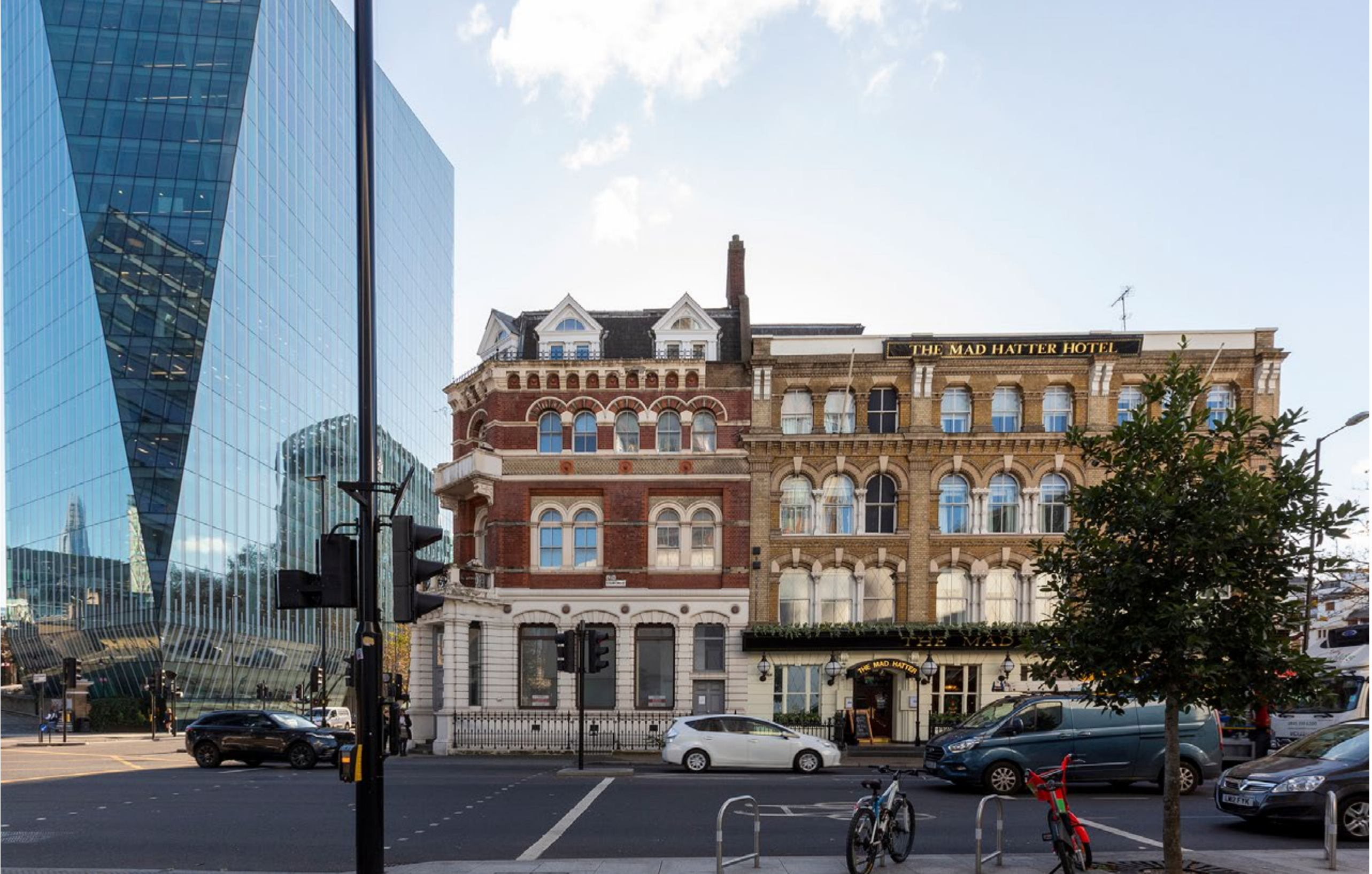
Right: Photograph of 1 and 3-7 Stamford Street - 2021
