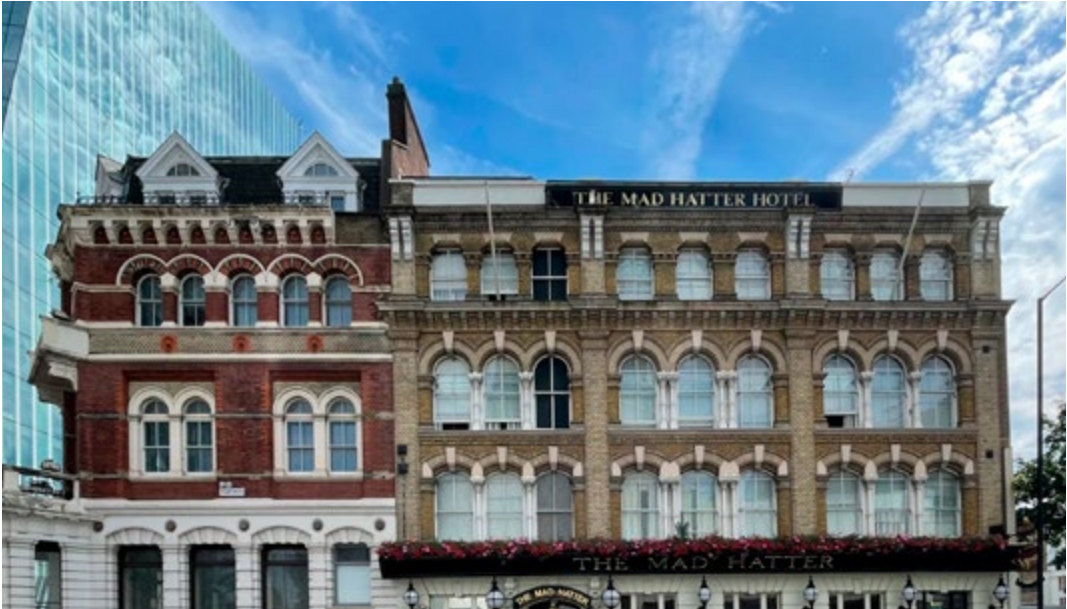
Top Left: 1 Stamford Street - Level 04 Bottom Left: 1 and 3-7 Stamford Street Northern Elevation Top Right: 3-7 Stamford Street Roof - Looking West Bottom Right: 3-7 Stamford Street Roof - Looking East
