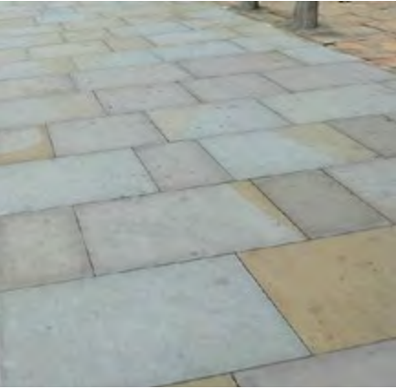
Yorkstone Slabs Sidewalks and base paving in public realm
