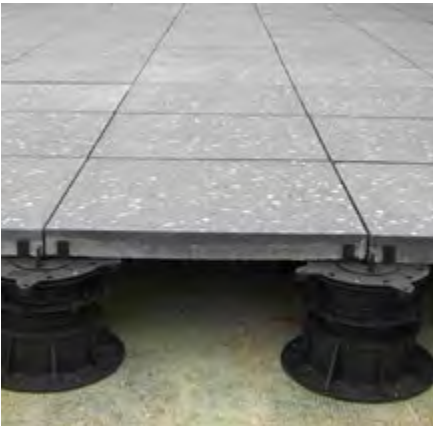
Composite pavers on pedestal system
