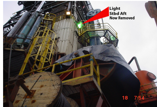
LOCATION OF LIGHT PRIOR TO FALL
