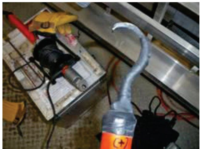
Phase Stick Hook Used to Check MCC
