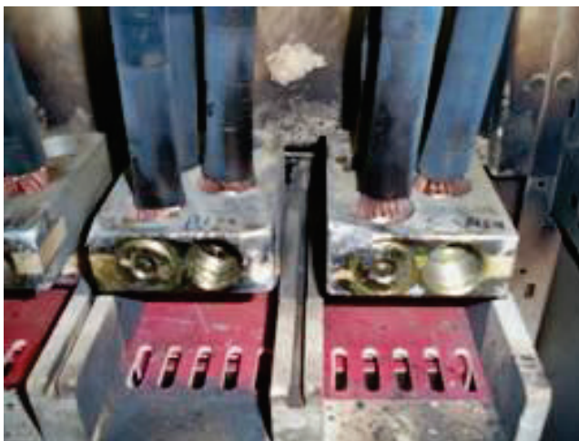
Phase B and C Lugs after the incident
