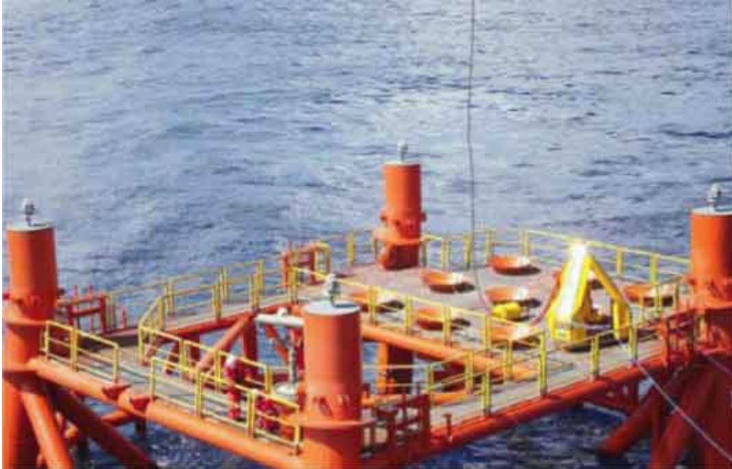
Platform jacket showing personnel lifting device and crane wire.
