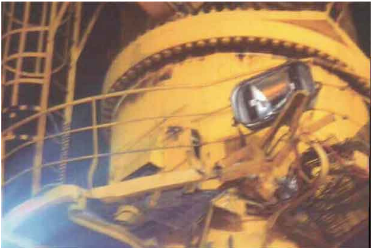
Damage to crane walkway and light caused by impact of swinging block
