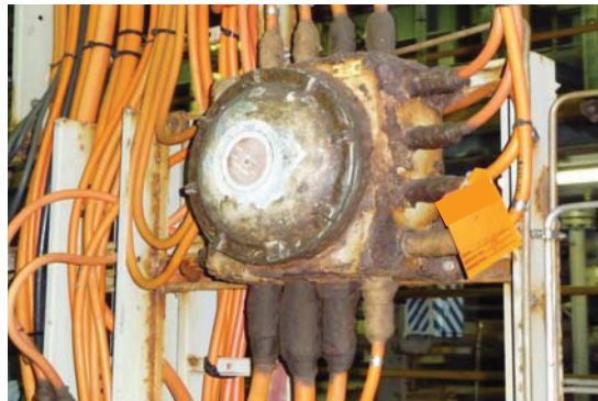
Photo 6 – Corroded Junction Box
