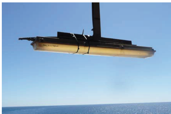
Photo 2 – Poorly Maintained Light Fitting in Process Area
