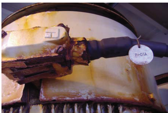
Photo 3 – Corroded Junction Box on Pump Motor
