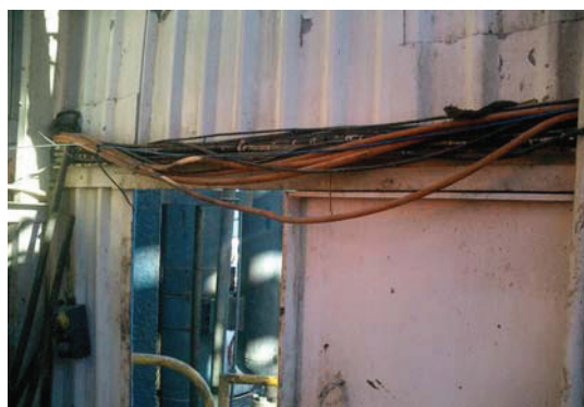
Photo 7 – Poor Dressing of Cables
