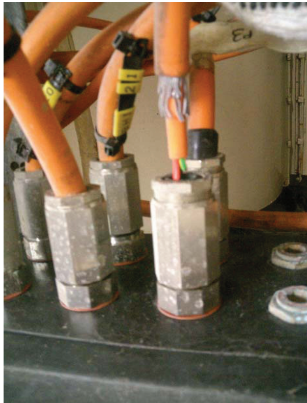
Photo 5 – Exposed Wiring (pulled out of gland)
