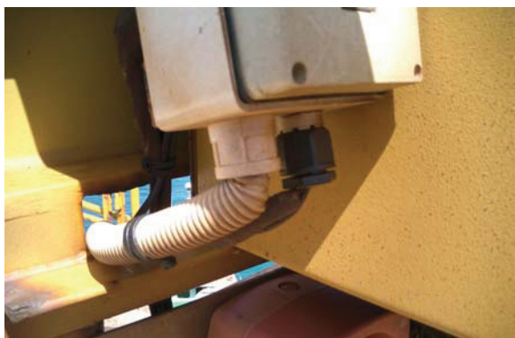
Photo 1 – Damaged Conduit and Exposed Wiring
