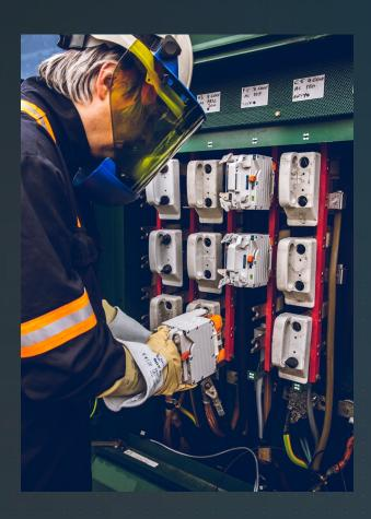
Bidoyng is a high-performance singleshot auto-recloser that rapidly restores supply after intermittent LV fault activity within the 3-minute regulatory outage period. Bidoyng's can dramatically reduce Customer Interruptions (CI) and Customer Minutes Lost (CML) figures whilst improving quality of supply to customers.
