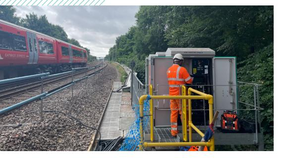
"On the West Coast Main line, Signet replaced the traditional LV power supply fuse protection systems to provide coordination and basic sectionalisation which was proving to be expensive and labour intensive and often resulted in long train delays and lost minutes. Signet solves this problem in a cost effective and controllable manner by automatically restoring power to affected signals and reconfiguring the system to isolate the fault."
