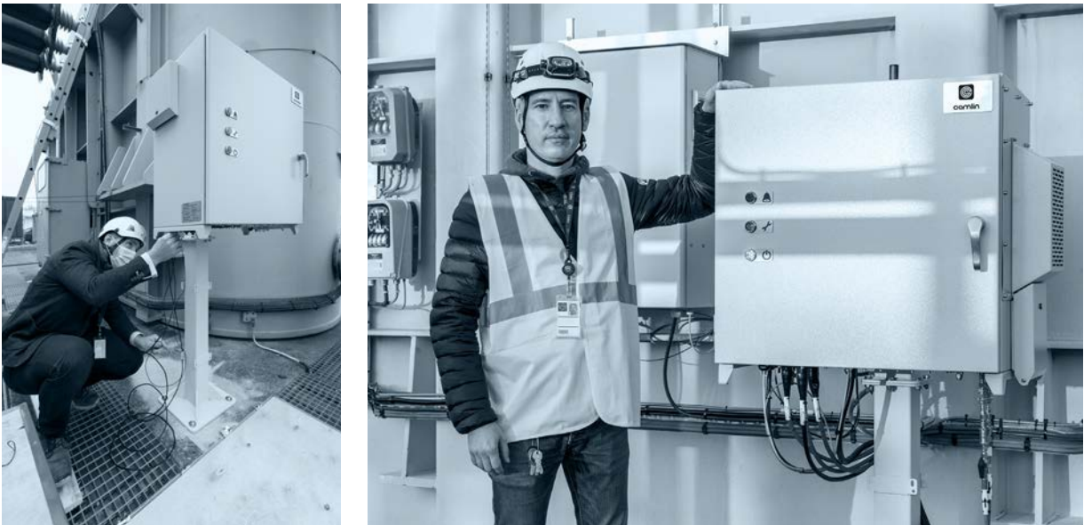
Customer Installation: T1-G5-INT3-TFC+TAM: TOTUS with DGA 5 Gas, PD and Bushing Monitoring on 3 bushings with Transformer Models
