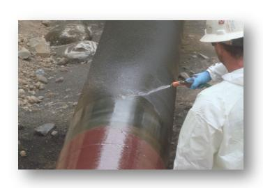
condensation. SP-4888® is also used for below ground corrosion control on pipe, piping assemblies, valve assemblies, pipe components and girth welds.
