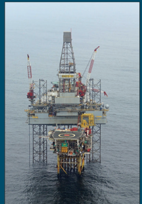
ENSCO 101 - Drilled the Tesla well
