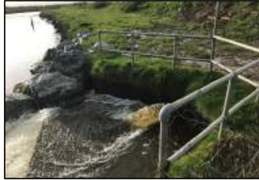
Plate 5-2 Existing headwall constructed from precast concrete and rock armour at the Rattoo pumping station.
