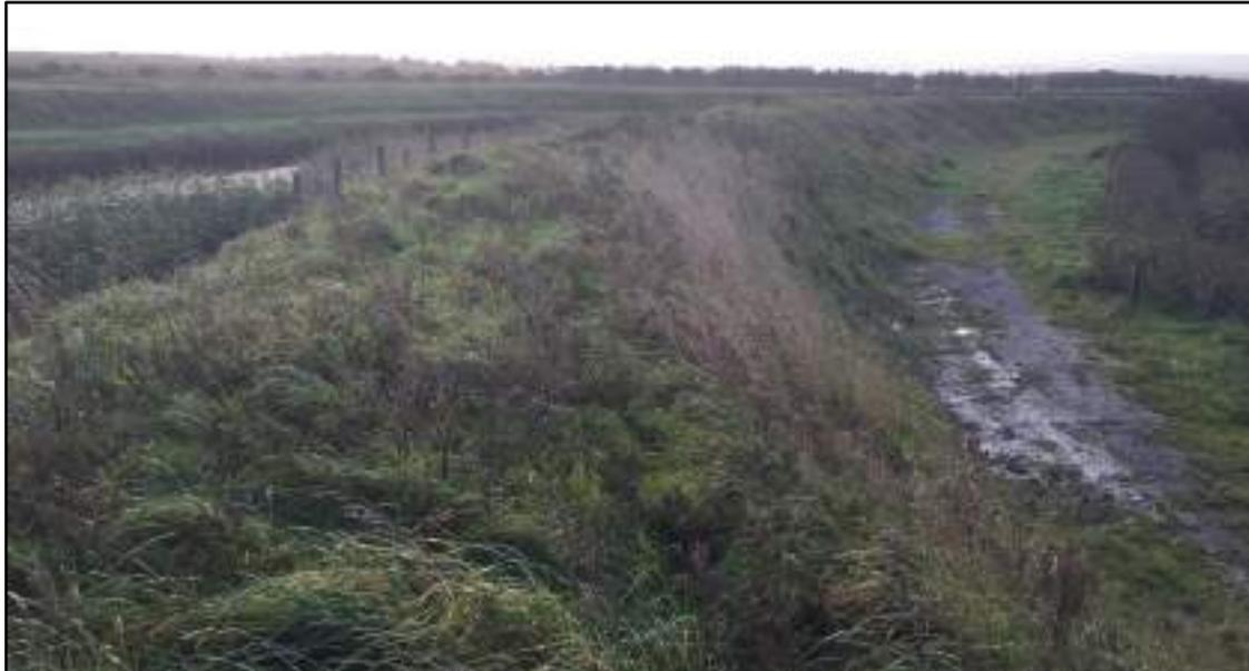
*Plate 3.6 Example of existing site access track (right) alongside an existing embankment (left). Such existing site access tracks will be used and upgraded where available.*
