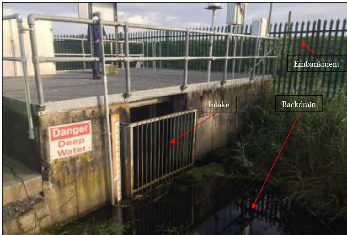
Plate 3.1 Example of existing electric pumping station within back drain, with flood defence embankment in the background.
