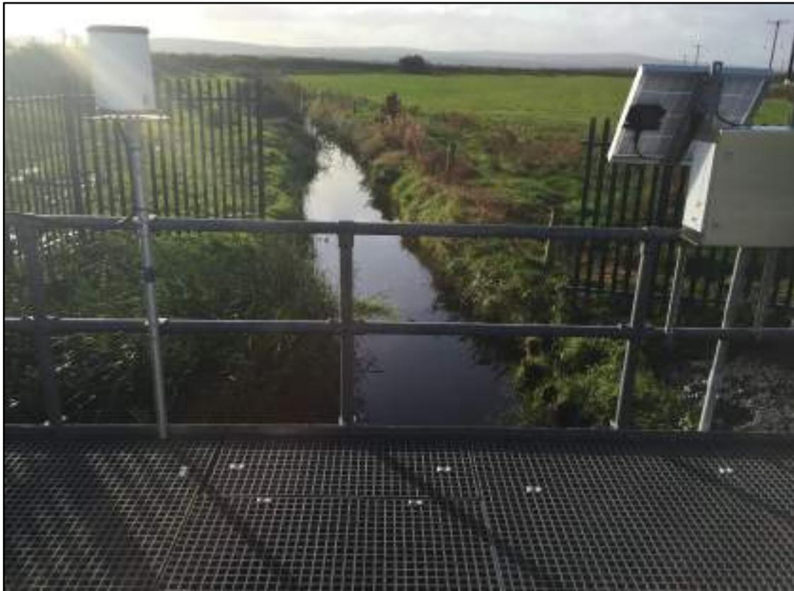
Plate 4.1 Example of existing back drain located on the landward side of the embankments. The back drains will be temporarily blocked off and the works area dewatered before installation of the proposed pump stations, as shown in the plate above
