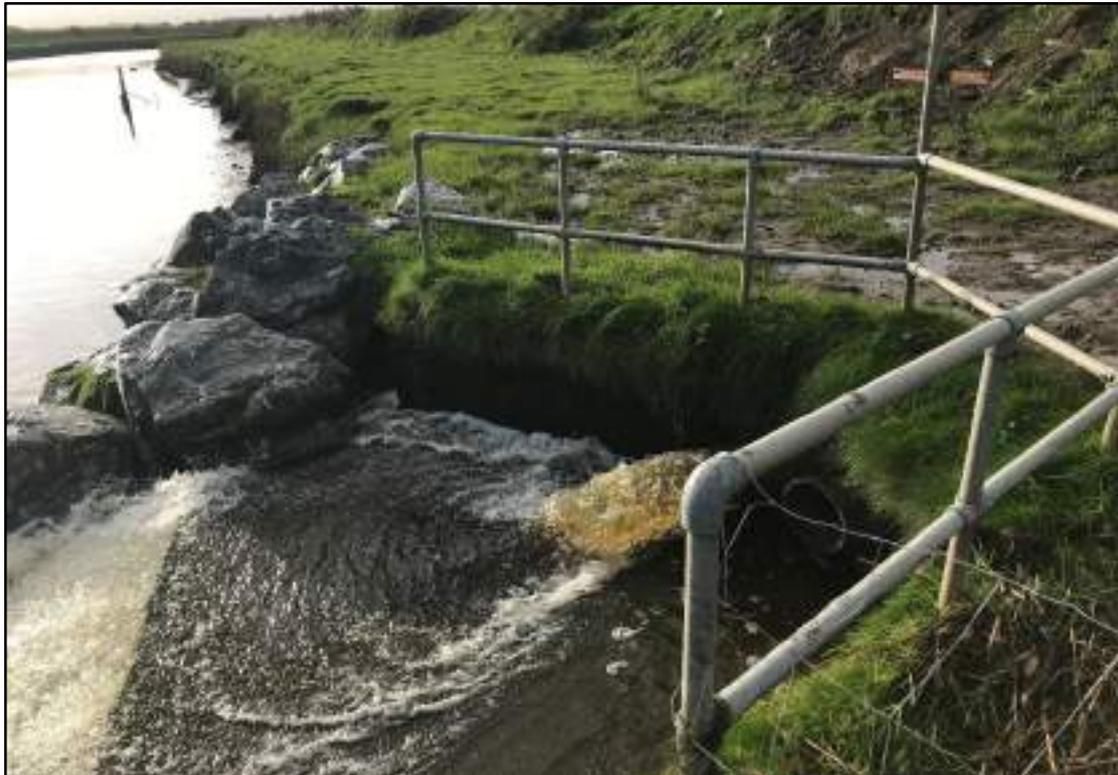
Plate 3.5 Example of existing outfall to the River Feale from the existing pump with rock armour surrounding the discharge to prevent scouring.
