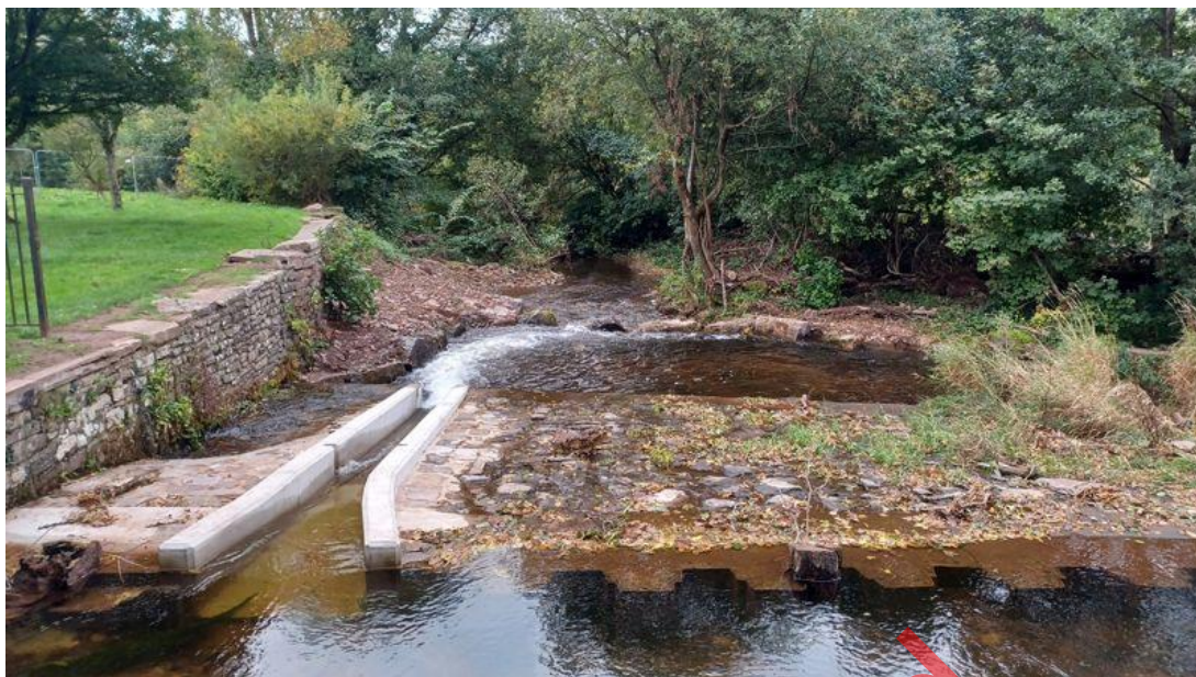
Figure 6-1. An example of a newly formed smolt chute through Brecon weir on the River Usk, designed by Fishtek. Whilst the required smolt chutes at Ness weir would be of a greater scale, the same fundamental design principles regarding inflow behaviour and attraction flow apply.
