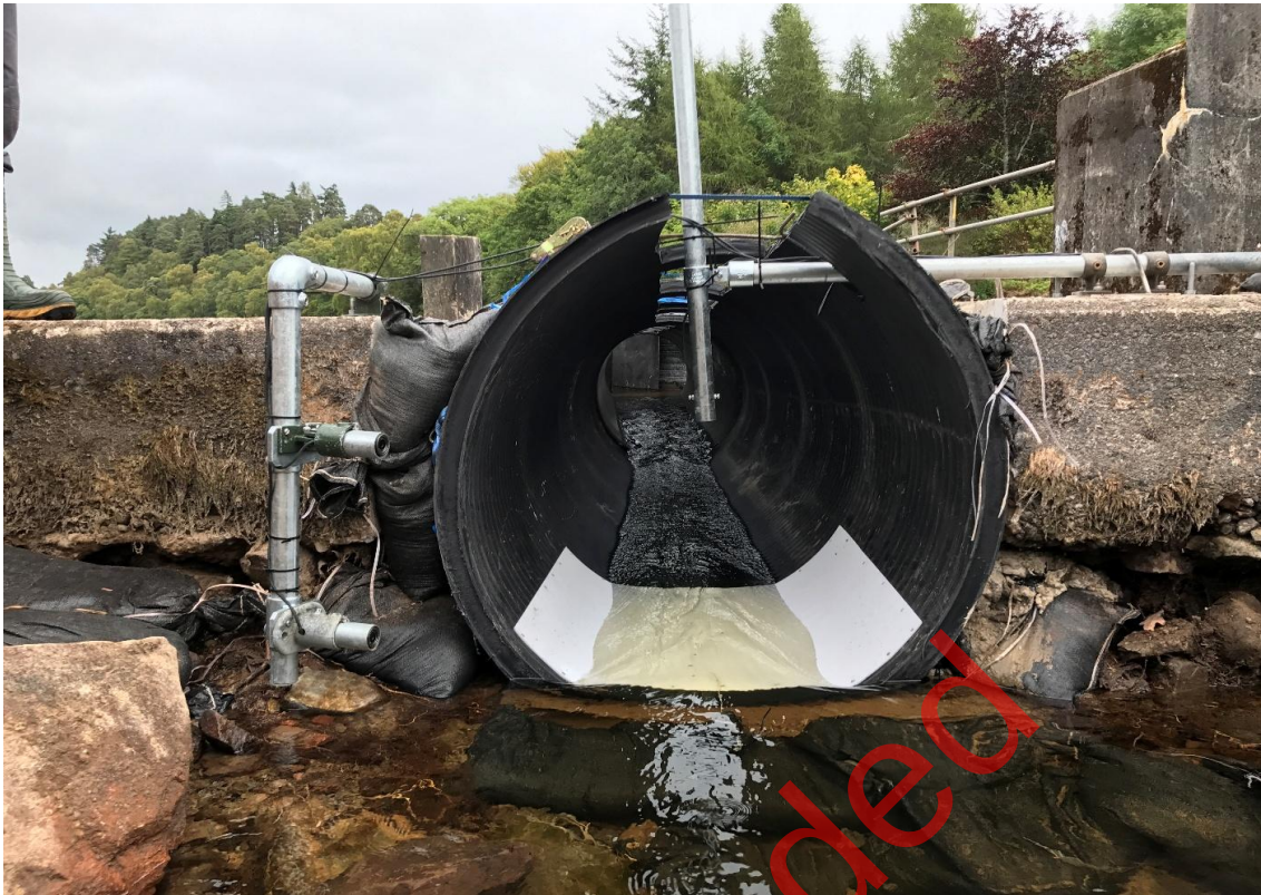
Figure 2. Photograph of the upstream exit from the fish pass lead-in channel, shown during construction under low loch water levels. Sideways and overhead gantries and white boards were included in the design to allow video camera monitoring of fish exiting the fish pass.
