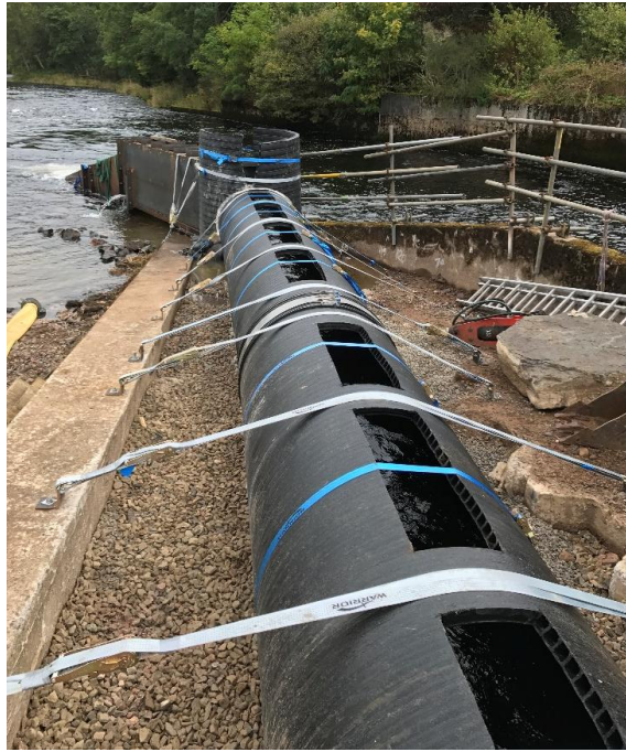
Figure 1. Photograph of the temporary fish pass installed at Dochfour Weir during the Scottish Canals piling repair works, facing downstream.
