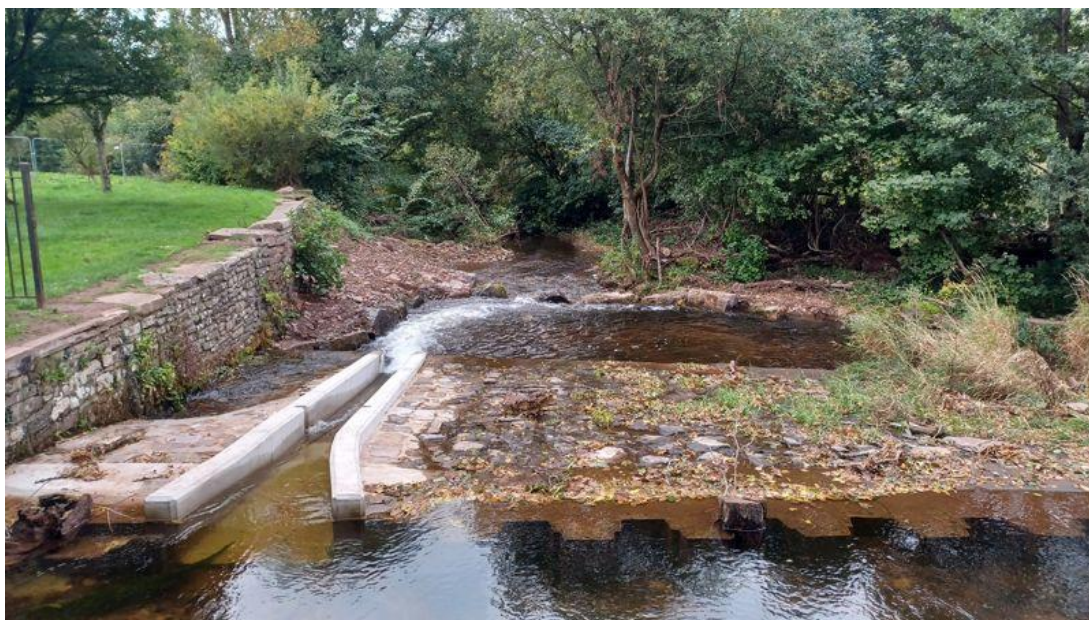
Figure 6-1. An example of a newly formed smolt pass through Brecon weir on the River Usk, designed by Fishtek. Whilst the required smolt channels at Dochfour Weir would be of a greater scale, the same fundamental design principles regarding inflow behaviour and attraction flow apply.
