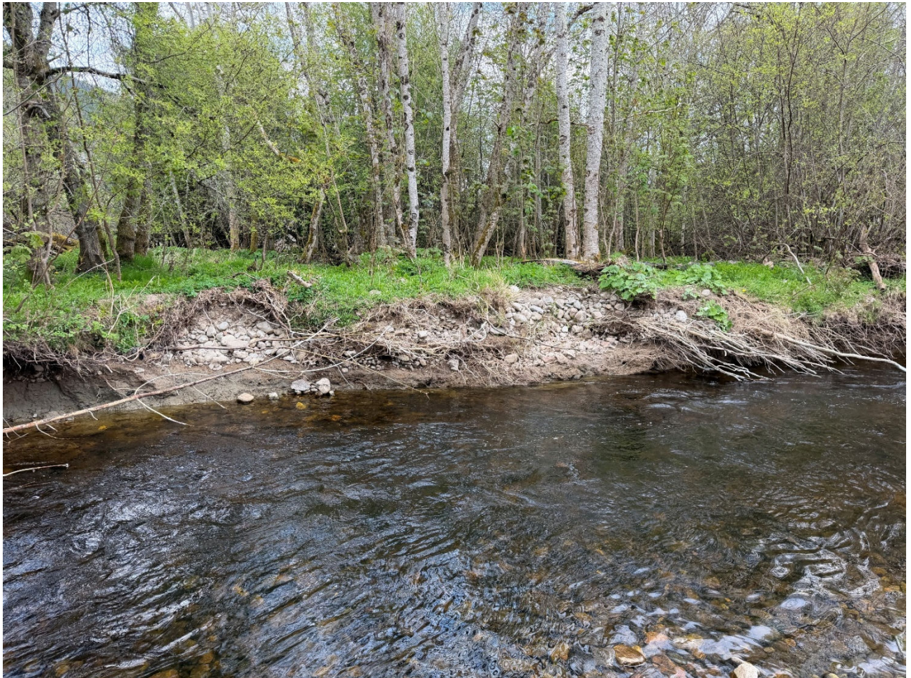
Figure 4 - Exposure of coarse sediment (predominantly cobble and gravel) overlaying a deposit of finer material (sand and silt) in an eroding channel bank within the proposed inundation zone but set back from the loch shoreline. This composite sedimentary character of the banks reflects the highly dynamic fluvial environment of the site, with continual changes of dominant geomorphic process (and, therefore, sedimentology at a particular location).
