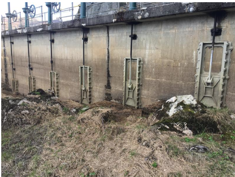
Figure 1. Fish pass inlet penstocks on the upstream face of Spey Dam shown during a period of reservoir drawdown. Individual penstocks are set at different invert levels and open and close automatically in a pre-defined manner in response to measured reservoir water levels.
