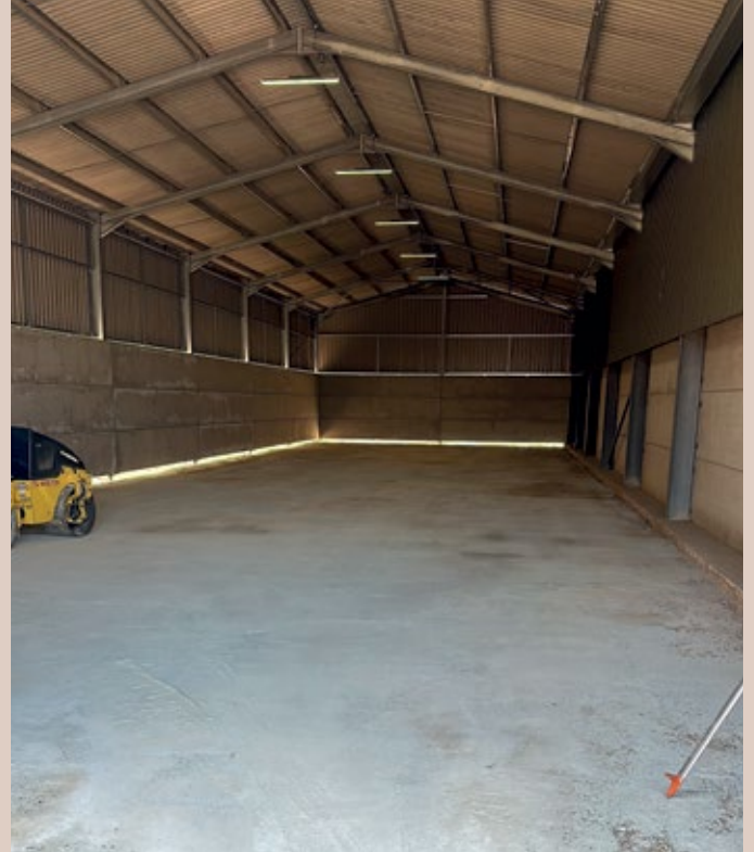
Prepping shed base before laying the floor
