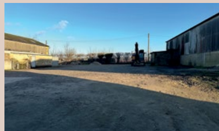
Concrete yard before
