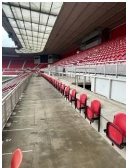
South Stand Accessible Deck
