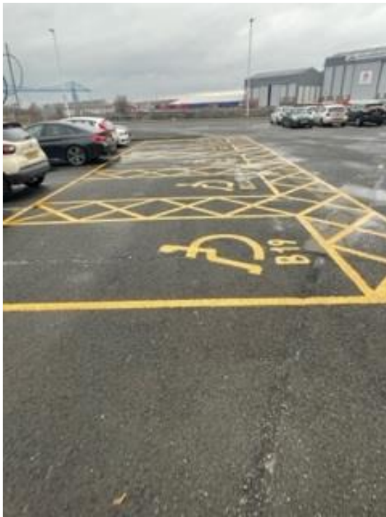
An Accessible Parking Bay
