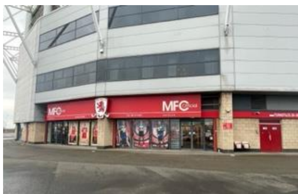
Retail Store Exterior
