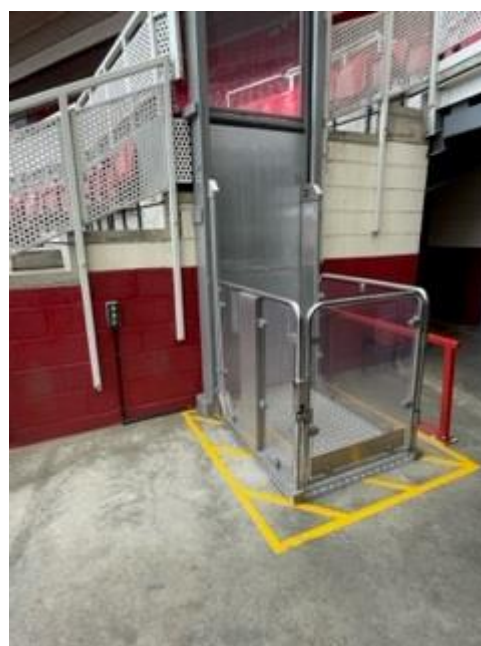
Lift to Visitor Accessible Deck
