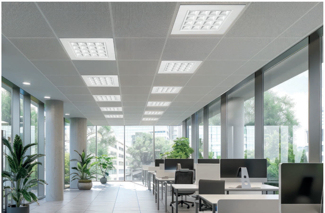
Offices and VDU-equipped environments.
