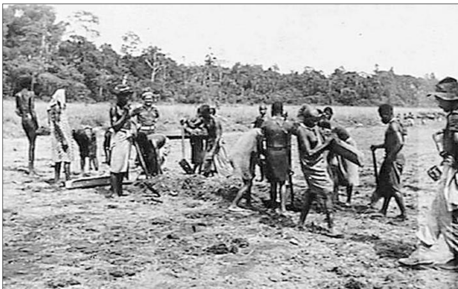
AWM 128792 - Construction of the airstrip at Hayfield, New Guinea, by pioneers of the 2/7th Australian Infantry Battalion with help of about 200 natives. 1945. Picture from John and Anne Moten
