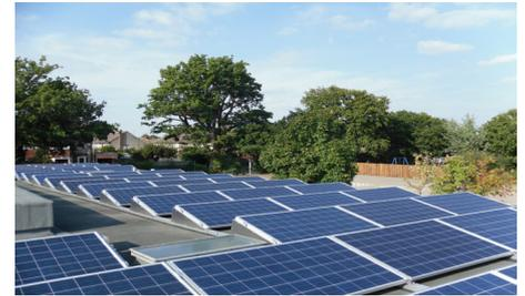
Home Farm Primary School has 50kW of solar panels installed on the roof, making the school self-sufficient in electricity.
