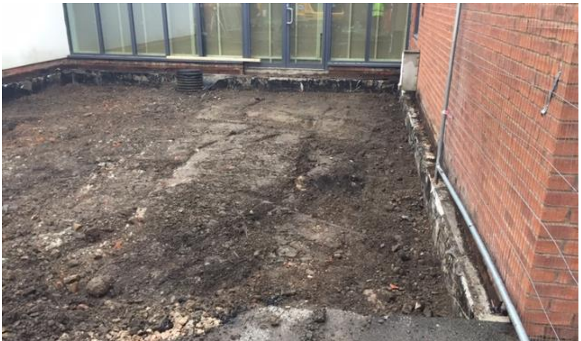
Courtyard area with slab removed
