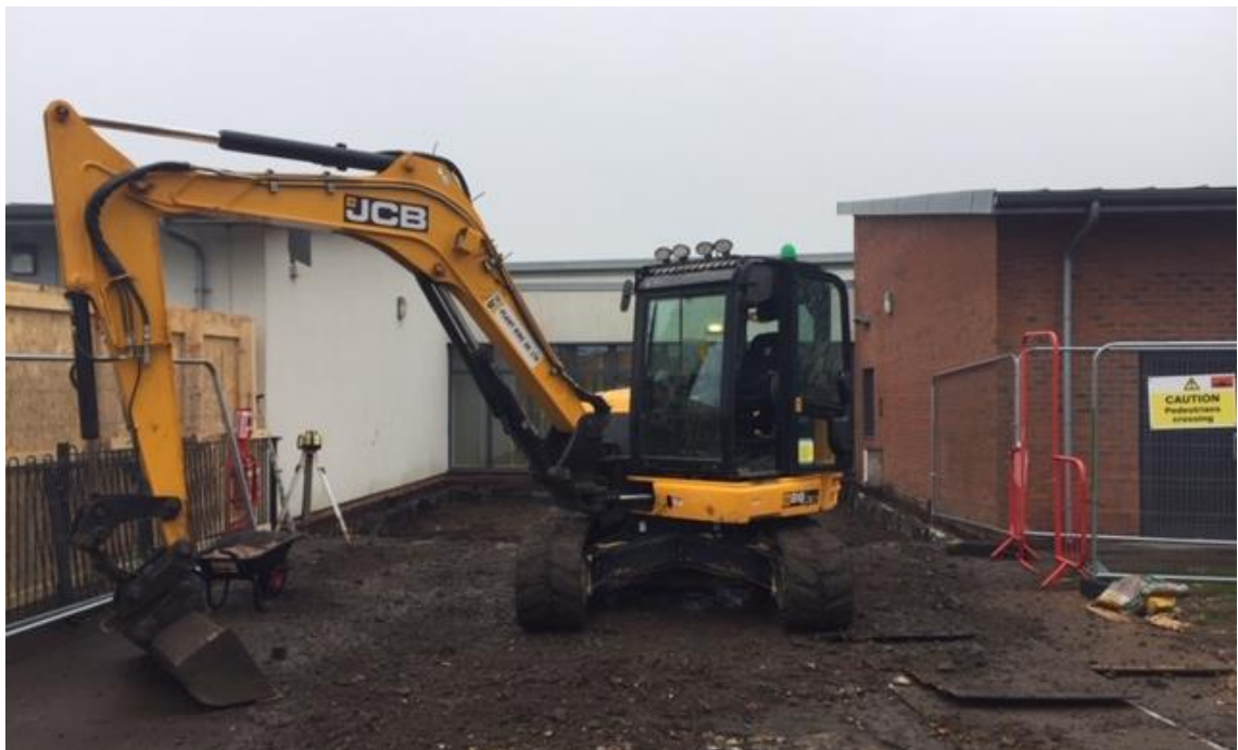
Infill classroom to courtyard area.
