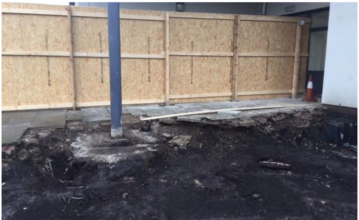
Exposed existing foundations to canopy
