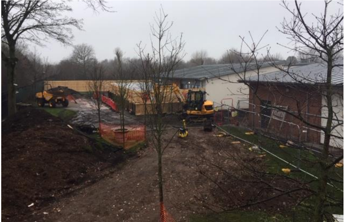
View across construction site from Site Accommodation
