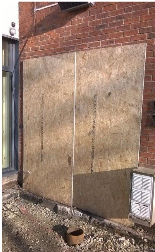
Boarding protection to Laundry Room window
