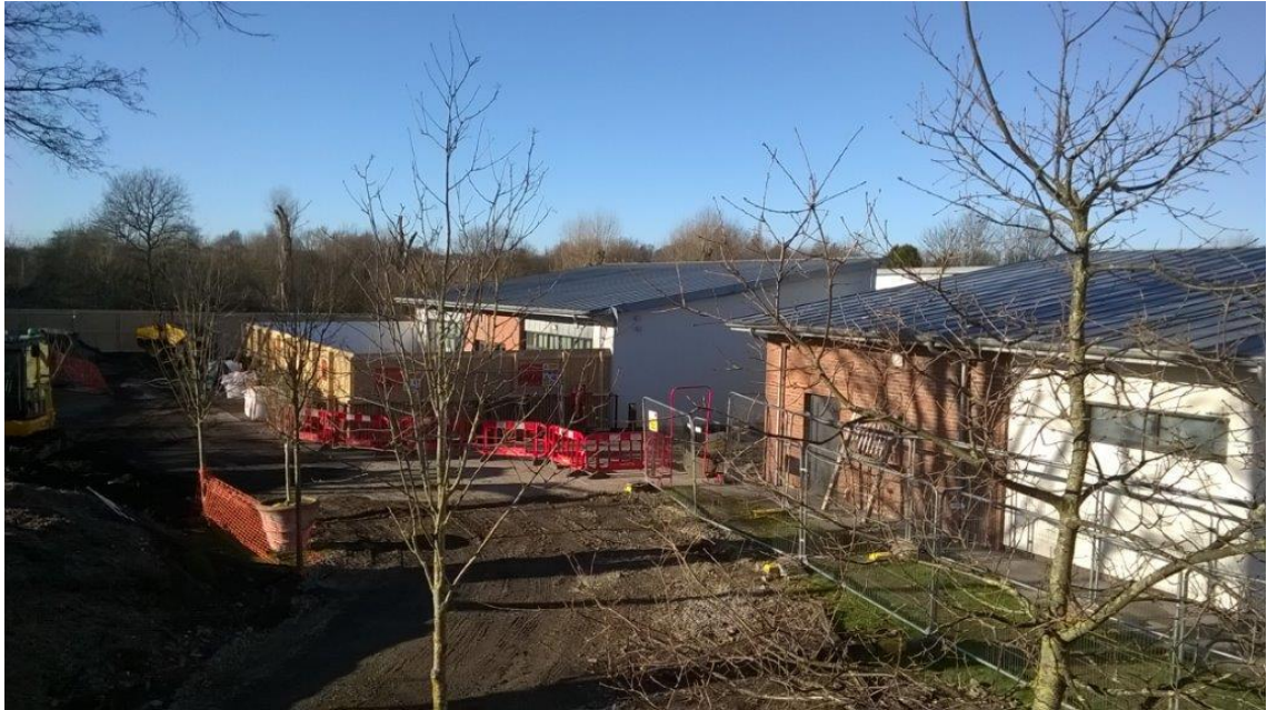
View across construction site from Site Accommodation
