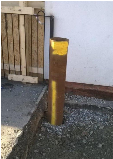
Steel Pile protruding above ground (awaiting test and cut down)
