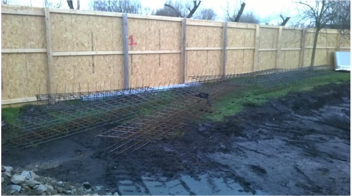
Steel Reinforcement cages for ground beams
