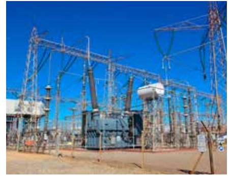
69/13.8 kV Substation
