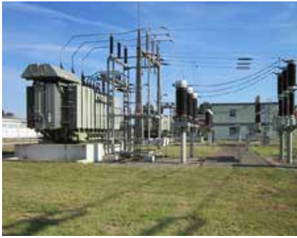
138/13.8 kV Distribution class substation at Utilities
