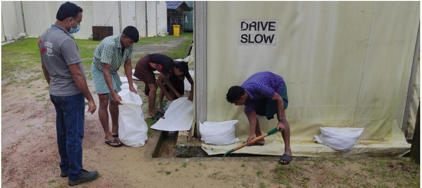
Drainage Cleaning at Balukhali Logistics Hub. Photo: Logistics Sector/Paul Karmoker
