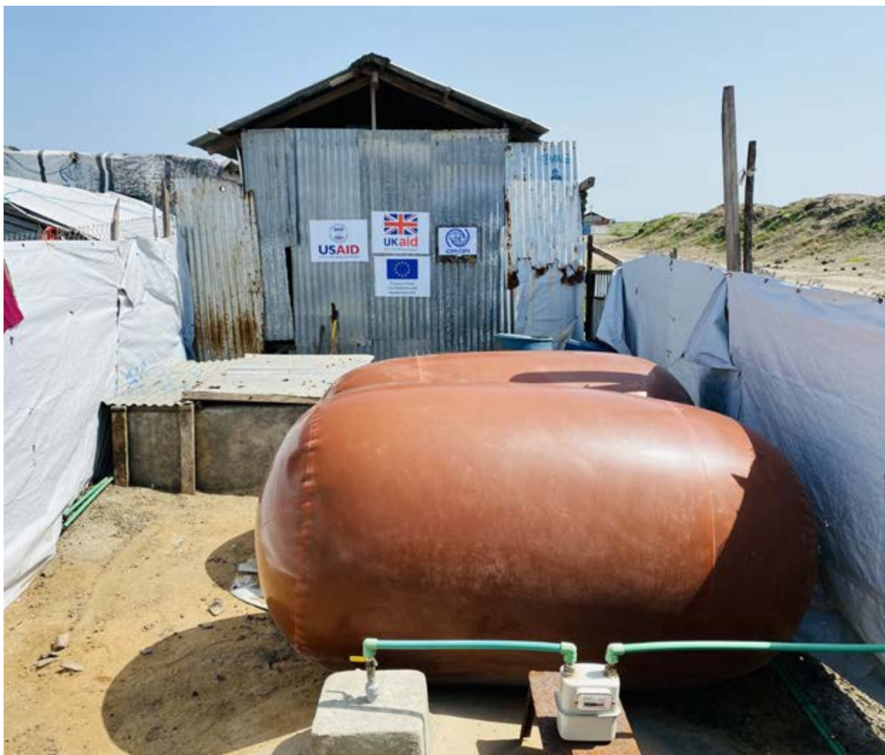
Gas storage balloons filled with biogas produced from treated faecal sludge at biogas site. © Oyugi Geophrey Owino/IOM
