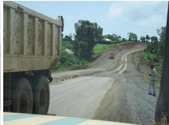
V. Mizan –Bonga Tarmac road under construction
