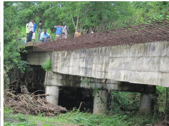
T. Akula Bridge under construction suspended – 2006
