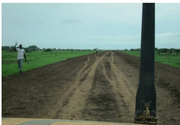
E. Metar Junction to Akobo Road under construction
