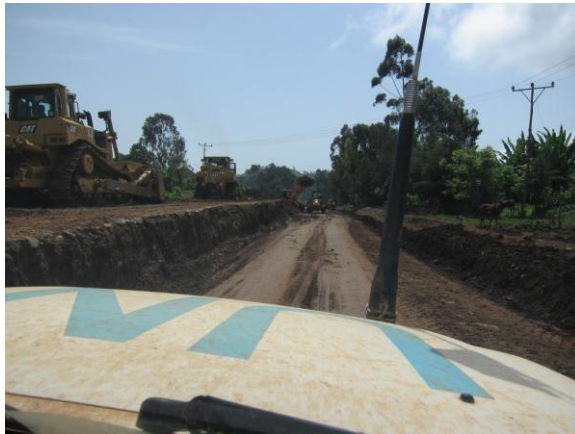
U. Mizan – Bonga Road under construction
