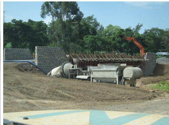
X. Bonga – Jimma: Bridge under construction
