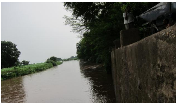
Gambella port: High water level expected in August month.
