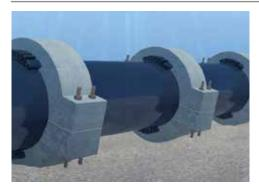
Fixing a sinker or thrust block to the pipe.
