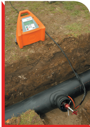
160mm Adjustable inlet Wastewater Saddle, offering an adjustable connecting angle of up to °12.
