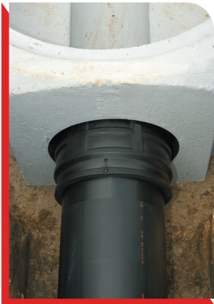
LightFit Coupler welded to a Manhole Adaptor
