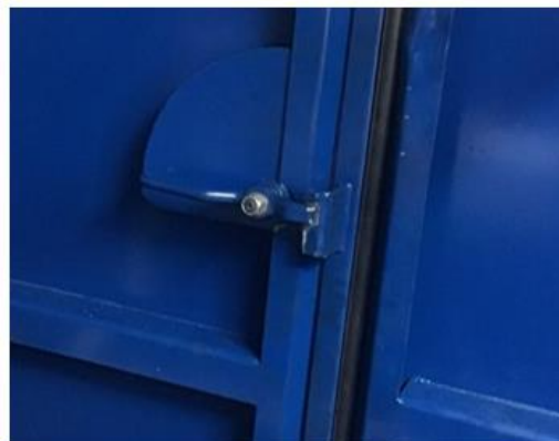
Locking device locks in the middle of the frame only, not to the top and bottom as required by the design standard
