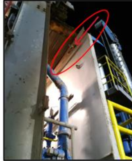
Figure 1. Drill Floor Deluge Line
