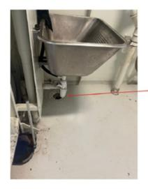
The H2S came from the drain under sink through the dry water trap.
