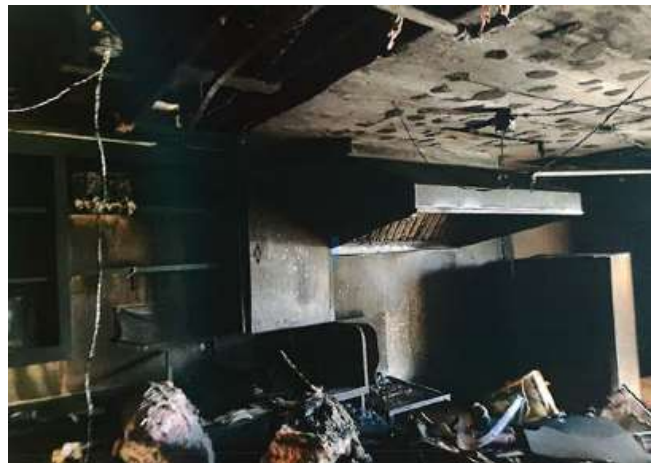
Fire spread to living quarters following hot work
