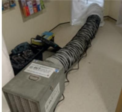
The works that required dust control were only able to be carried out at certain times each day so that the speed of setting up and taking down the dust extraction system including barriers was key to making the project a success.
