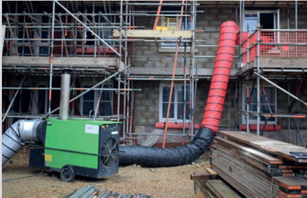
The 150Kw, 110V heater was sited externally with flexible ducting taking the heat into the building. Using several lengths of ducting to target different spaces simultaneously enabled rapid drying of multiple spaces. By forcing a flow of clean dry heat into the site, and through the positive pressure created by this method, the heat was evenly distributed throughout the building and thereby removed the moisture so successfully that no additional dehumidifying equipment was required.
