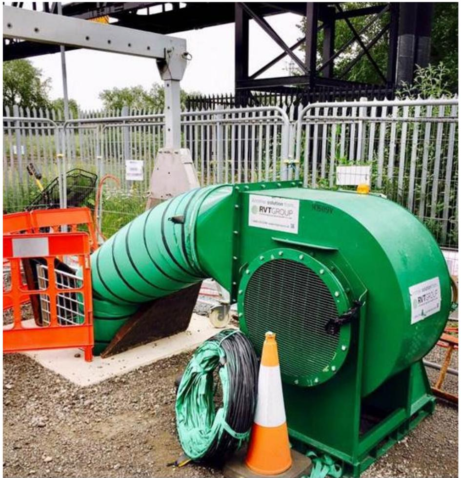
The 450 CF (Centrifugal Fan) chosen to drive the air is capable of generating airflow of 20,500m<sup>3</sup>/hr so was ideal to force a supply of fresh air through ducting into the furthest end of the sewer tunnel. In addition, the positive pressure created by the fan ensured contaminated air was continuously replaced.
