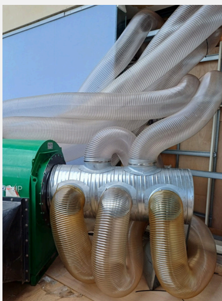
VENTEX® Centrifugal Fan 600S situated outside of the store
