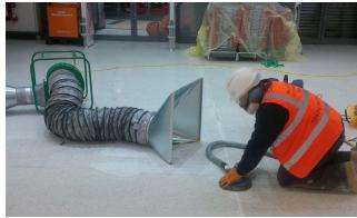
The CF 200P can be connected to any RVT filtration unit, as pictured.
