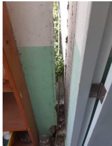
Figure 72 - Subsided extension
