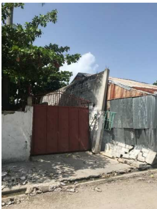
Figure 42- Building 25 boundary wall
