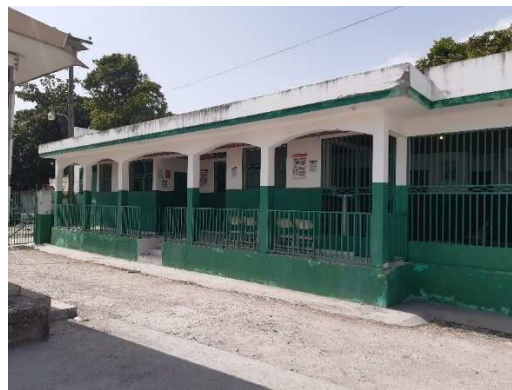
Figure 26 - Area of building 13 that could not be accessed
