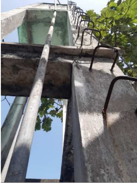
Figure 8 - Building 3, concrete water tower
