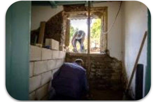
Small Repairs for Host Families
