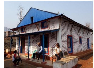
Load Bearing stone masonry in mud mortar; Location Sunkoshi Rural Municipality-06, Sindhuli, 2018 – ©HRRP
