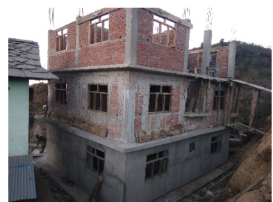
Reinforced Cement Concrete Framed, reconstruction Umakunda rural municipality, Ramechhap, 2017– ©HRRP
