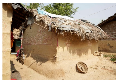
Flood protection. The basis of the walls is surrounded by a mud layer, which is cyclically eroded and repaired. Terai, 2016 – ©Marie Schuiten
