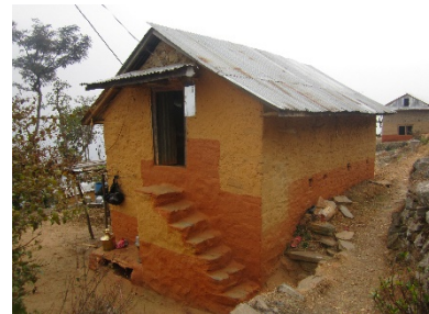
Stone in mud mortar house, with clay plasters, Kavrepalanchok, 2018.—©HRRP
