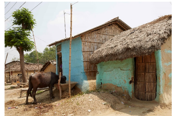
Bamboo walling and thatch roof, Terai, 2016 – ©Marie Schuiten
