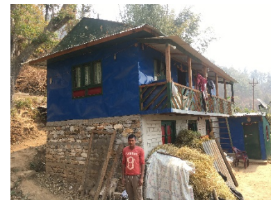
Hybrid structure, Timber and CGI fencing on masonry ground floor, Molung, Okhldunga. ©HRRP
