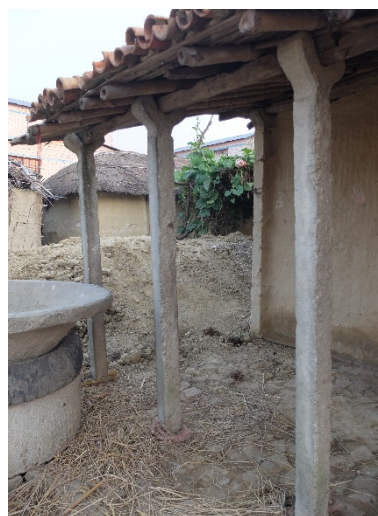
Floods protection. RCC post, Terai 2022 – ©CRATERRE
