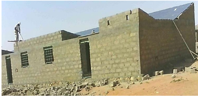
Ongoing construction of permanent shelters in Burao, Togdheer.
